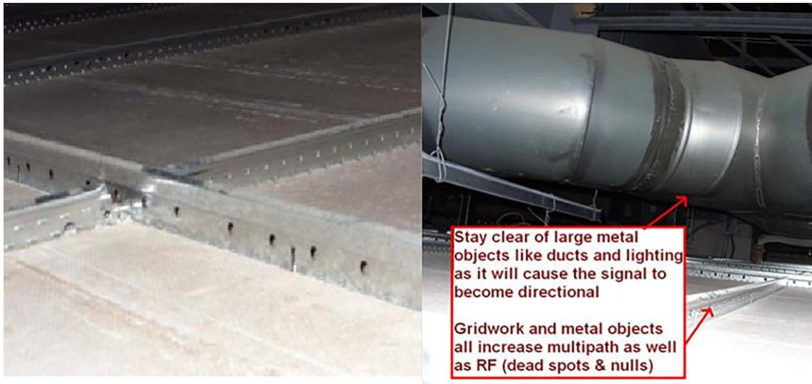
Figure 15. Installing the AP above ceiling tiles: pick an area clear of obstructions, avoid ceiling clutter
